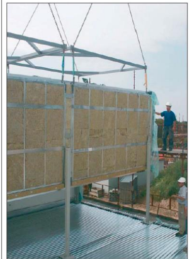
Fig 17. Installation of modules with recessed corners around SHS columns (courtesy of OpenHouse AB)
