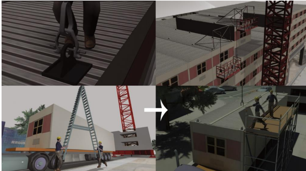
Fig. 5. Evaluation of construction operation scenarios: (a) proposed pop-rivet system for connections and lifting of modules, (b) use of scaffolding
