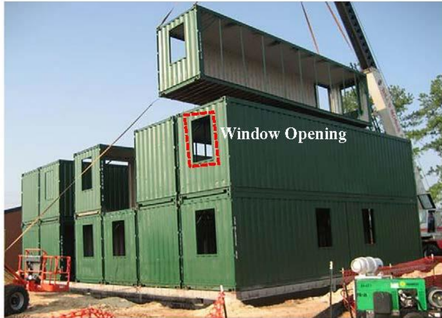
(a) Residential building
