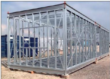
Fig 10. Corner-supported module
